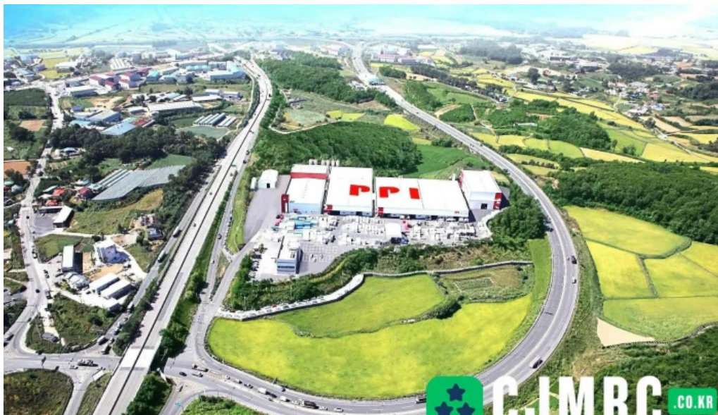
Ppi pipe jeonce
